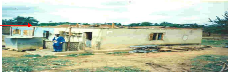
Plate 4.1: Roof Blown-off
