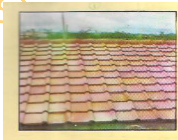
Plate 2.5b: Roof constructed with Tile
