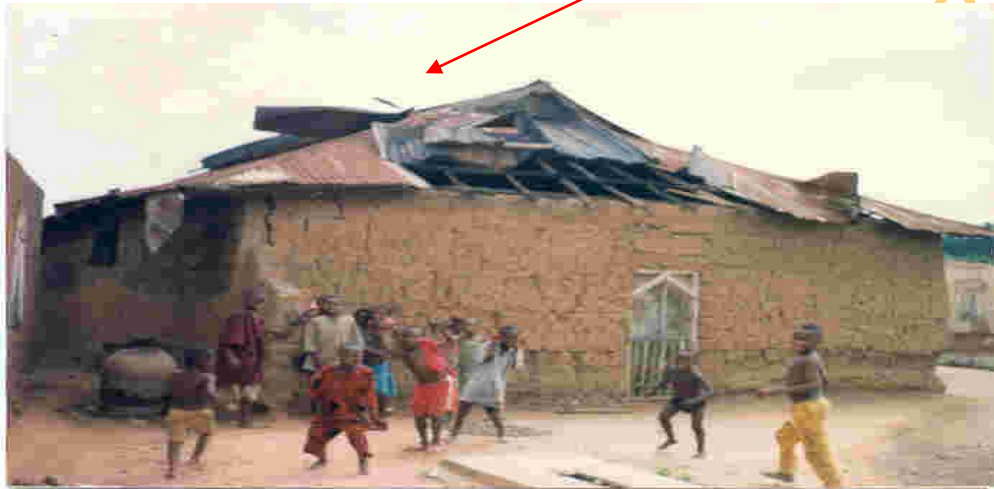
Plate 4.2: Sheet Removal
