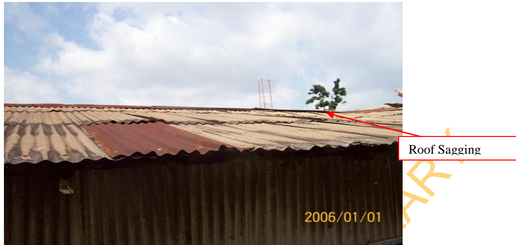
Plate 4.10: Roof Sagging
