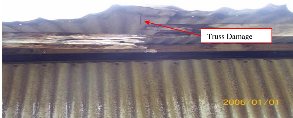
Plate 4.6: Truss Damage
