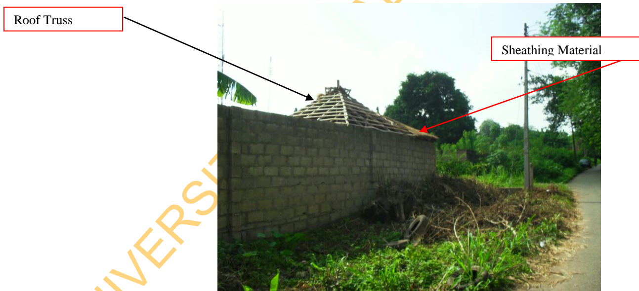
Plate 2.1: Roof Assembly Showing Truss and Sheathing
