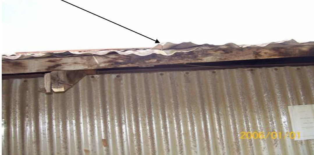
Plate 4.3: Nail Withdrawal
